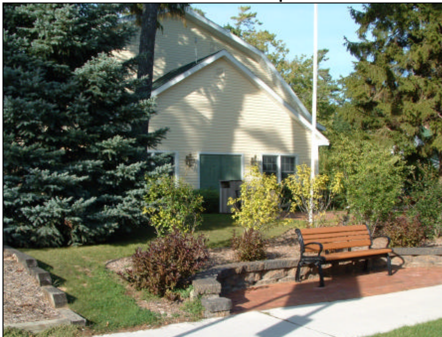
Photo 4-1 Glen Arbor Township Hall
