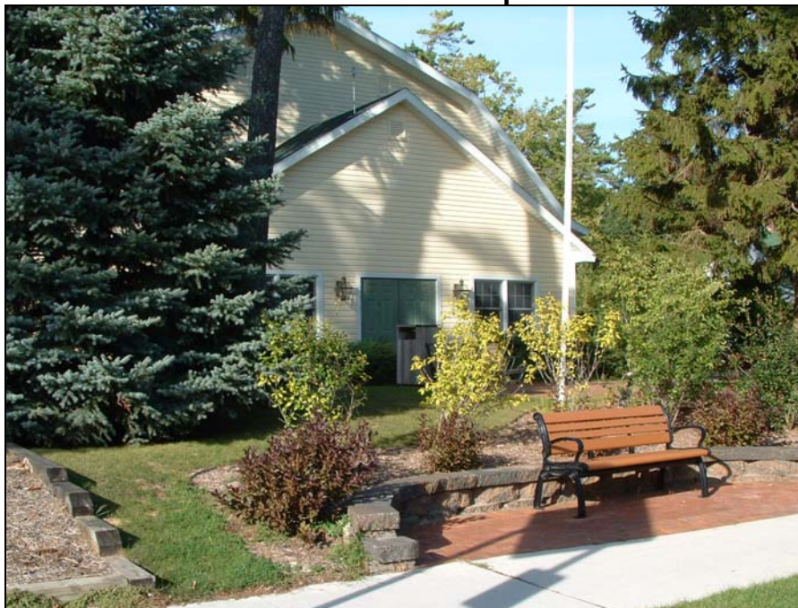
Photo 4-1 Glen Arbor Township Hall
